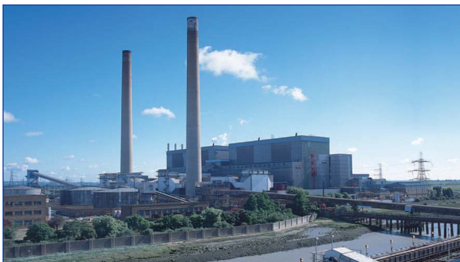
Figure 15: RWE Tilbury plant, UK: Dedicated biomass
